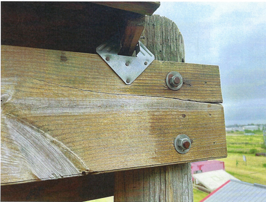
Board is cracked from the end to the other side of the post.
