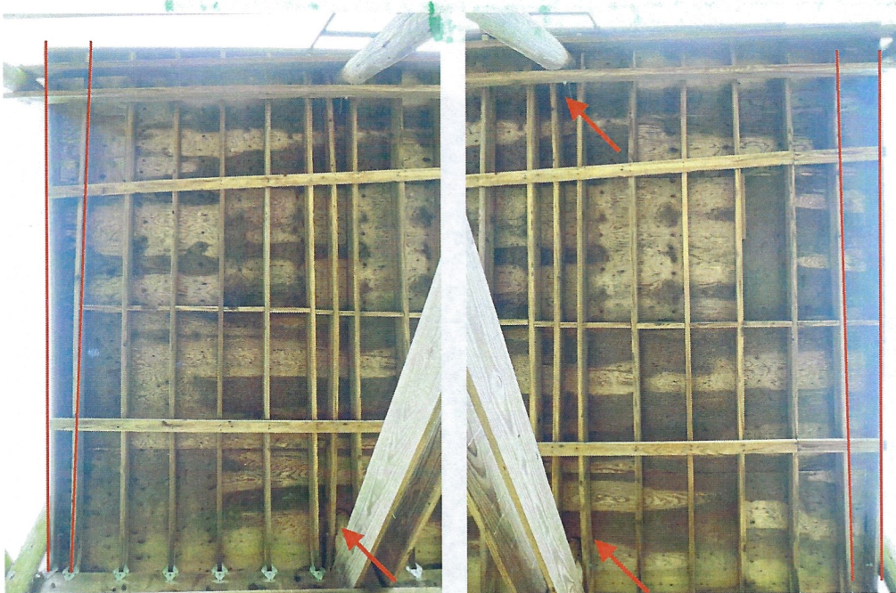
The roof decking was holding moisture. Joists are not all flush and those in the center appear bent around the vertical posts (arrows).
