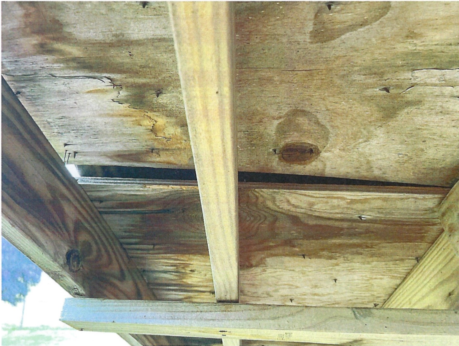
A section of the roof is warped and raised. The decking appears to be rotting where it has lifted.
