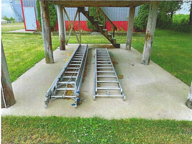
Concrete foundation is in good shape, no cracking or damage observed.
