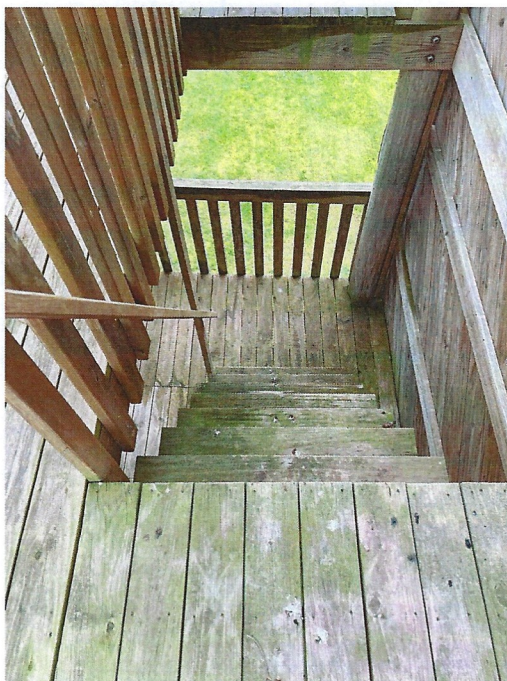
Stairs from the second to third level have an excessive rise per OSHA standards.
