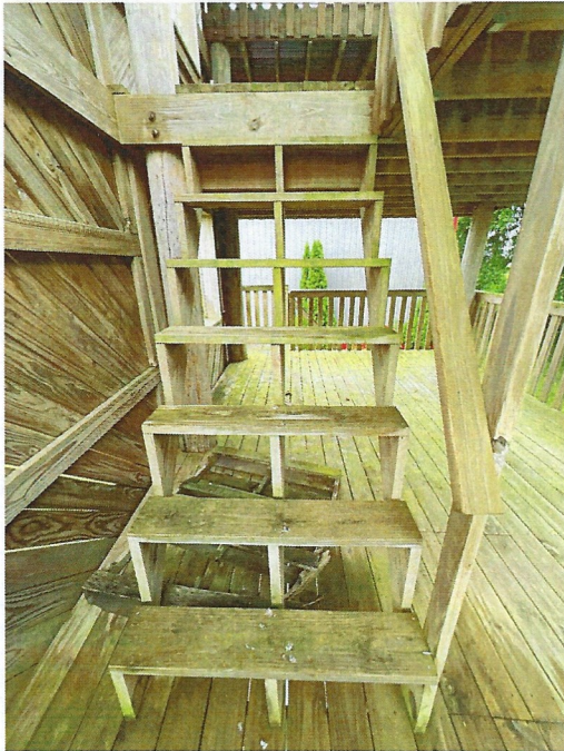
Stairs from the second to third level have an excessive rise per OSHA standards.
